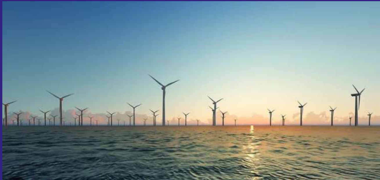
Tampnet has installed 4G coverage at the Hornsea One windfarm, making it fully digital
